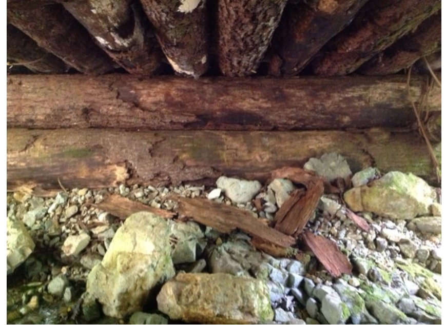
Left Bank Abutment when facing downstream
