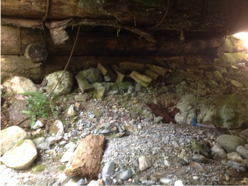
Right Bank Abutment when facing downstream
